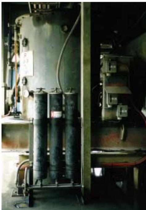
Servicing can be done while the crusher is still operating and is typically done on a three monthly basis with oil samples taken to monitor trends. An added benefit of the systems had been an increase in oil life of more than 800%. Some crusher systems have been operating for three years with oil analyses still returning good results.
